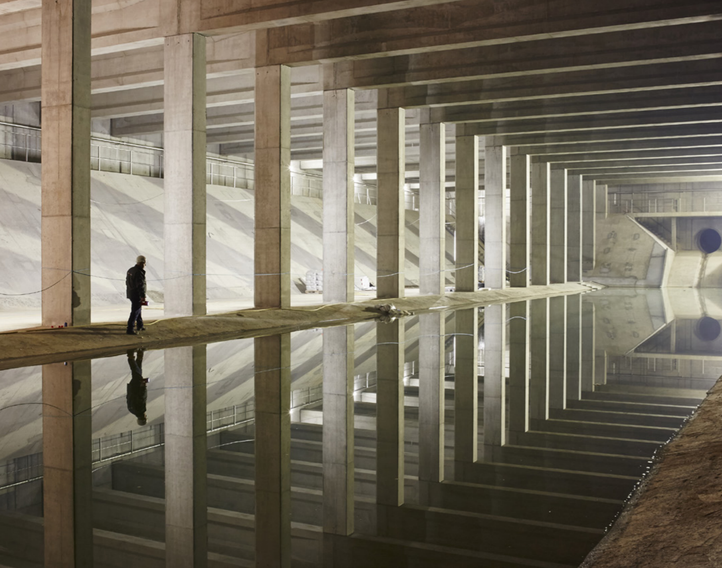
Water reservoir Simmering, © City of Vienna
