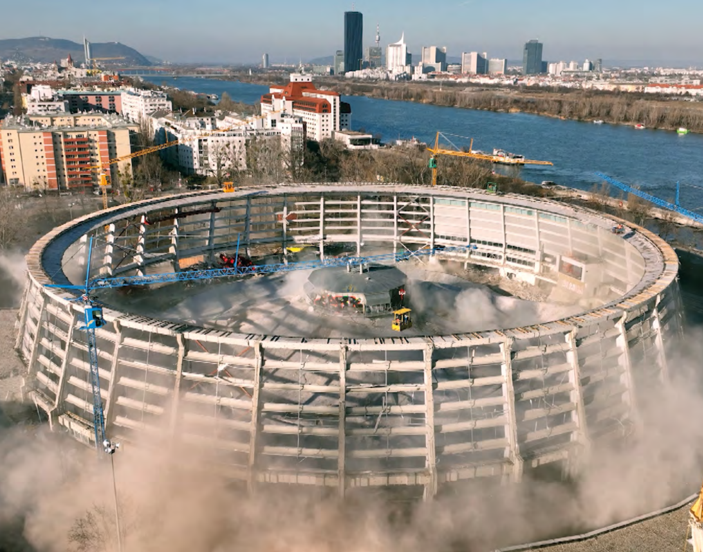
Demolition of the Ferry Dusika stadium © Jakob Gramm/MA 51-Sport Wien
