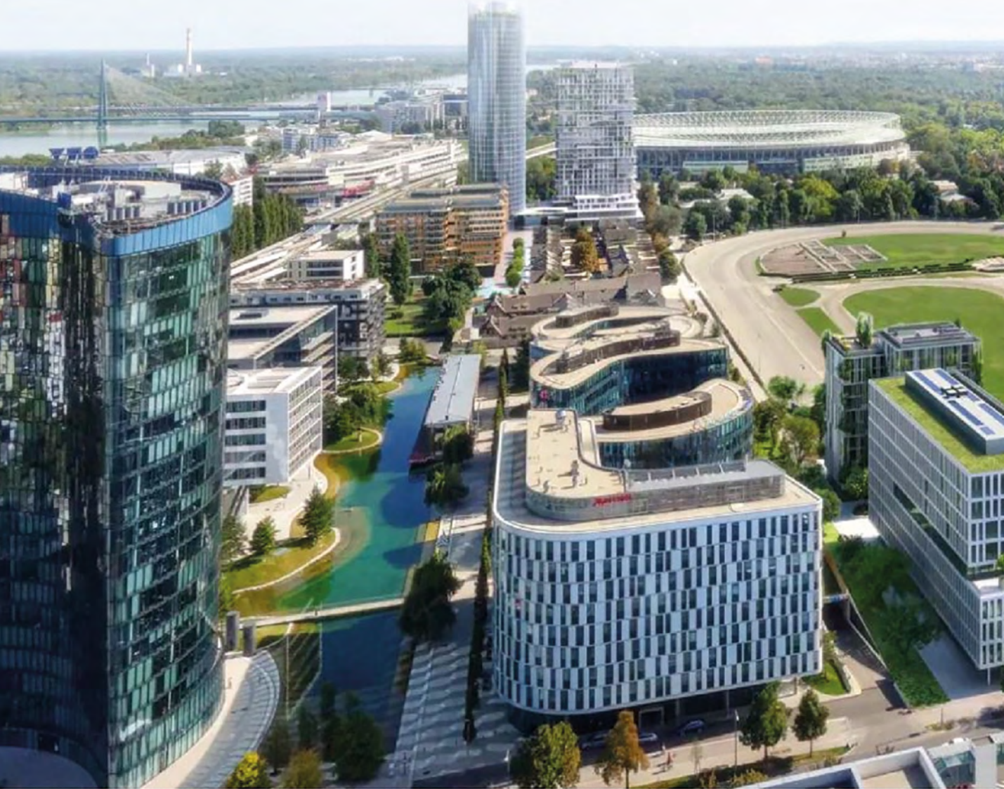
Generating green energy, storing it counter-cyclically and distributing it intelligently in the Viertel2 development © Value One / Office Le Nomade
