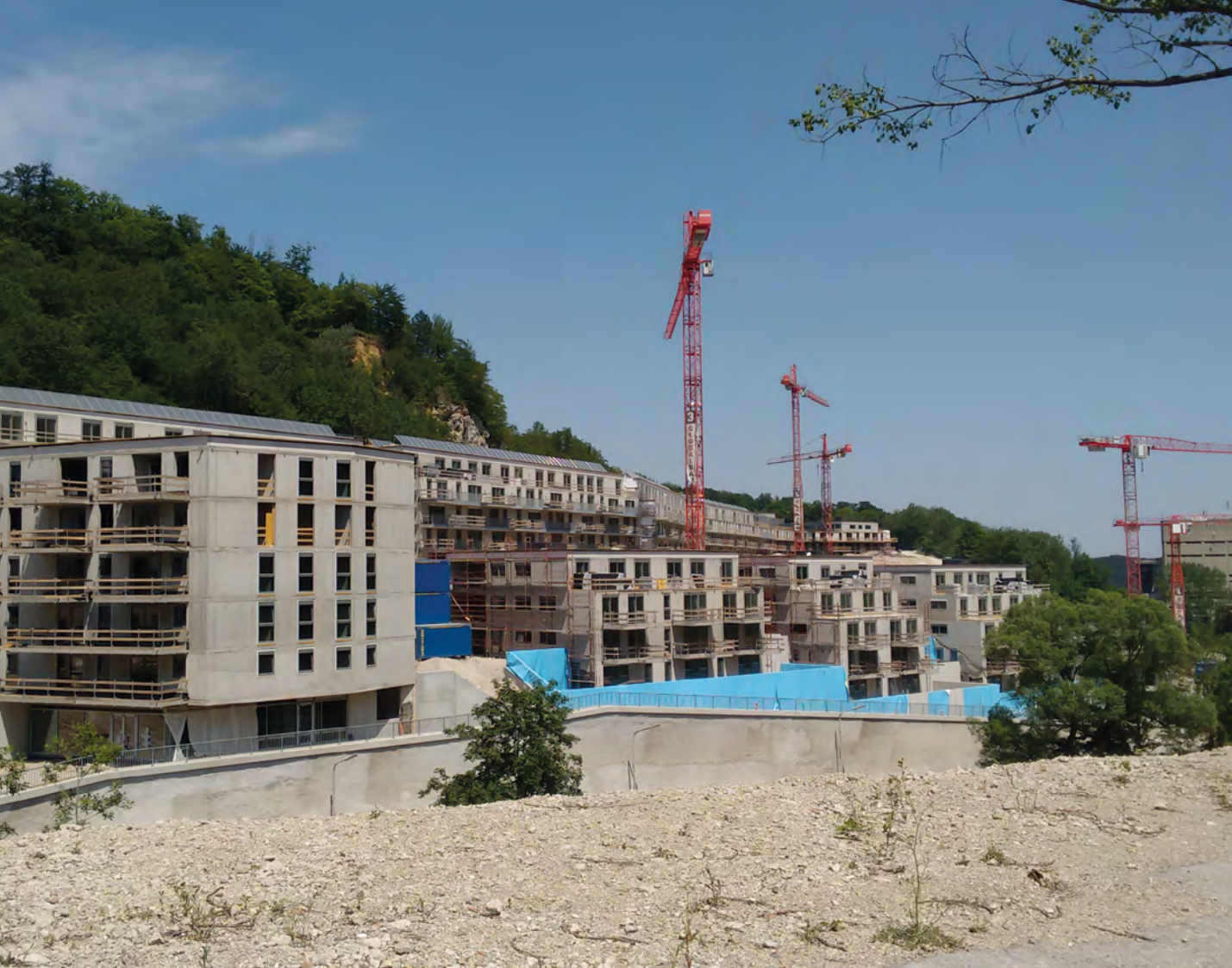
Construction of the Waldmühle Rodaun housing development © Ailura, upload.wikimedia.org/wikipedia/commons/9/90/20150705_Wohnanlage_Waldmühle_Rodaun_133035127.jpg
