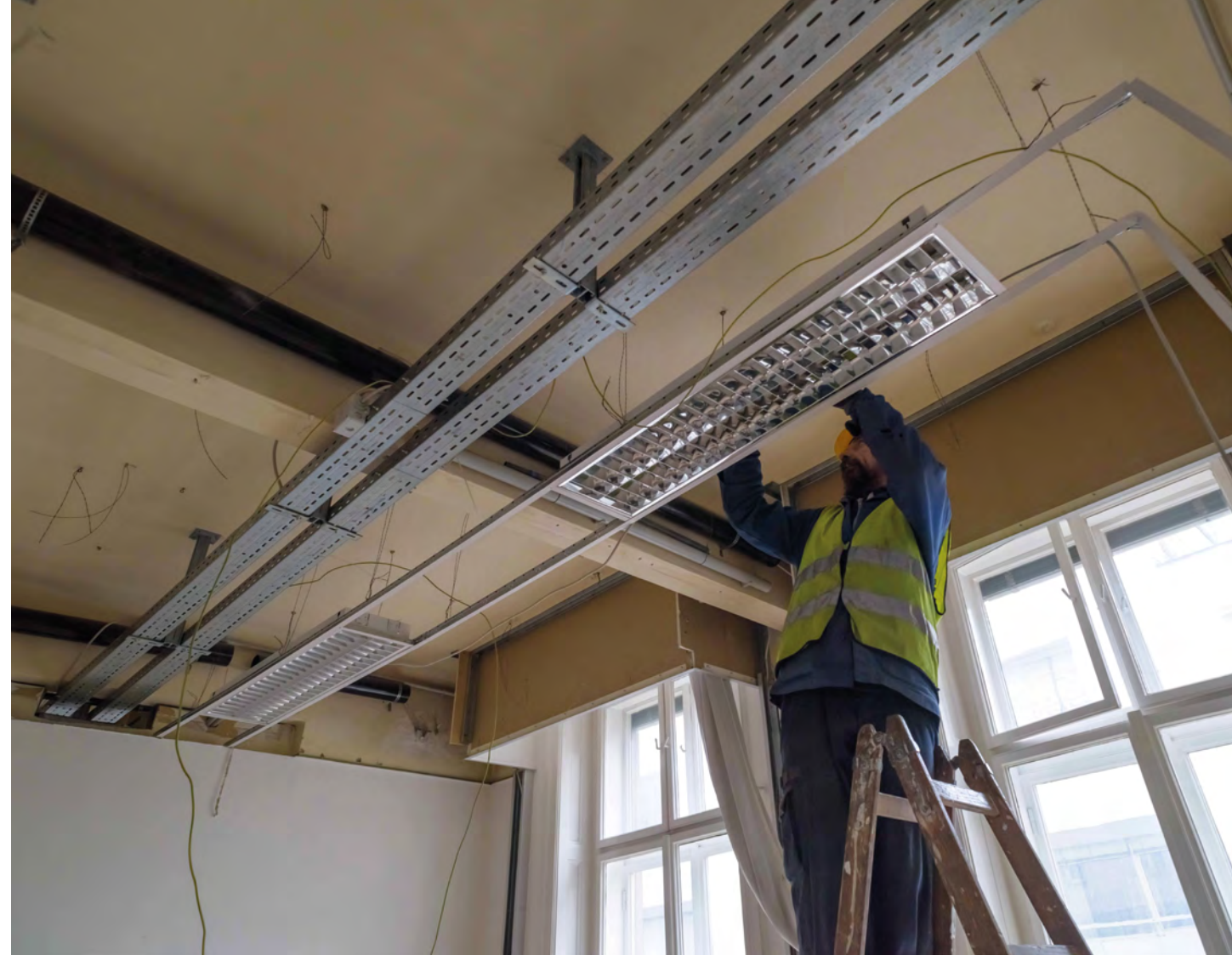
Separated material and component removal at the former Vienna Energy Centre © Harald A. Jahn
