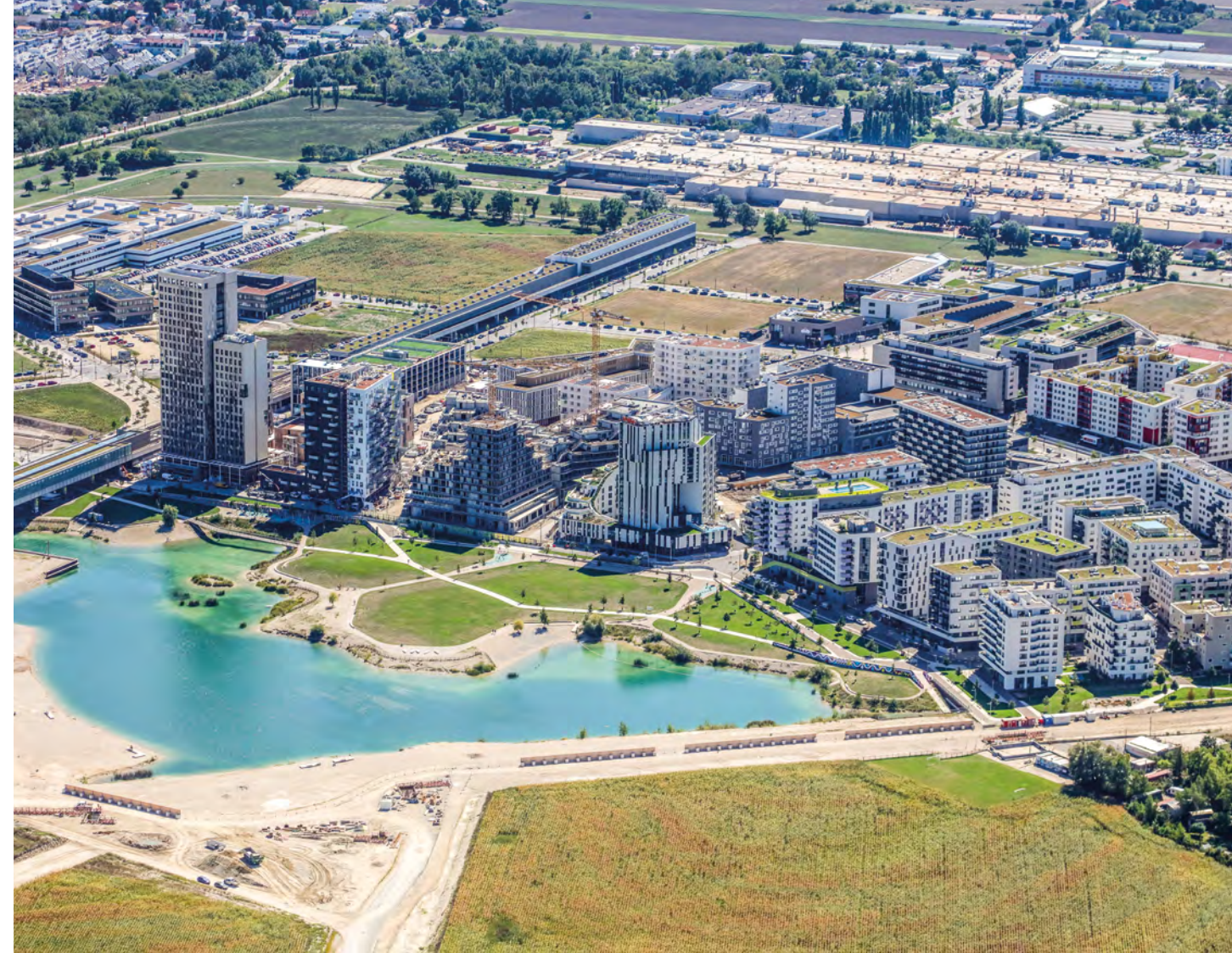
Gravel from the excavation of the lakeside area is used for in-situ concrete production © Christian Fürther | MA 18
